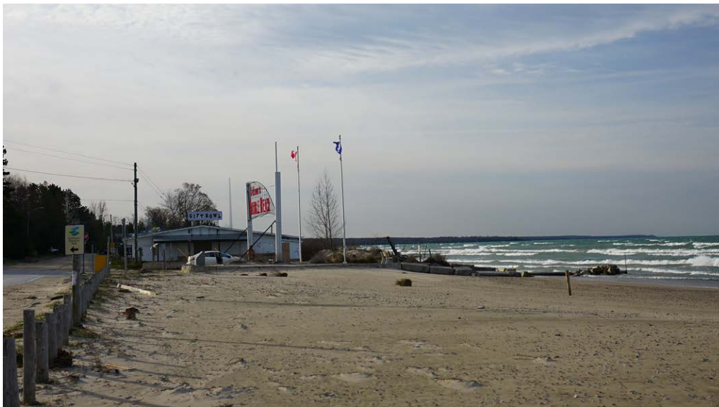
Figure 2.8 Failed Block Promenade at Sauble Sign, November 19, 2020
